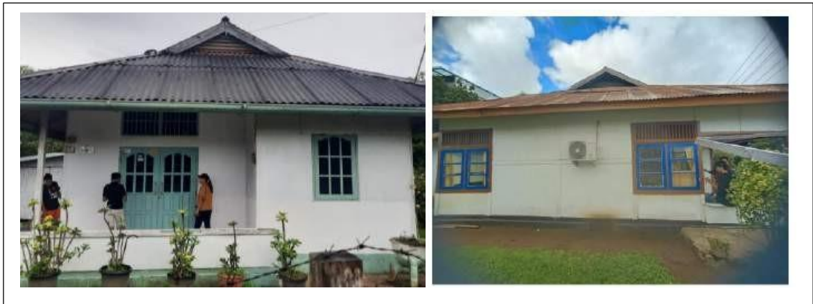
Figure 5 Roof model of houses built during the Dutch colonial era in Merauke. Both using gable dutch type
