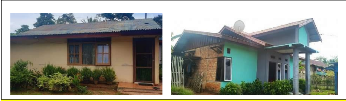
Figure 6 Rumah Kancingan with a terrace and without a terrace. House on the left was Rumah Kancingan without a terrace and the right was with a terrace.
