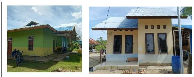
Figure 3 The Roof Shape of Rumah Kancingan built in 2000s.
