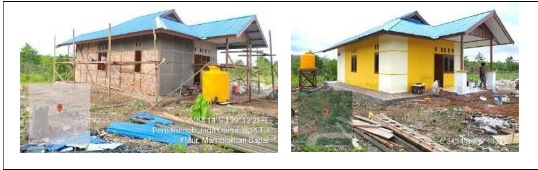
Figure 1 Rumah Kancingan before (on left) and after the construction process(right)
