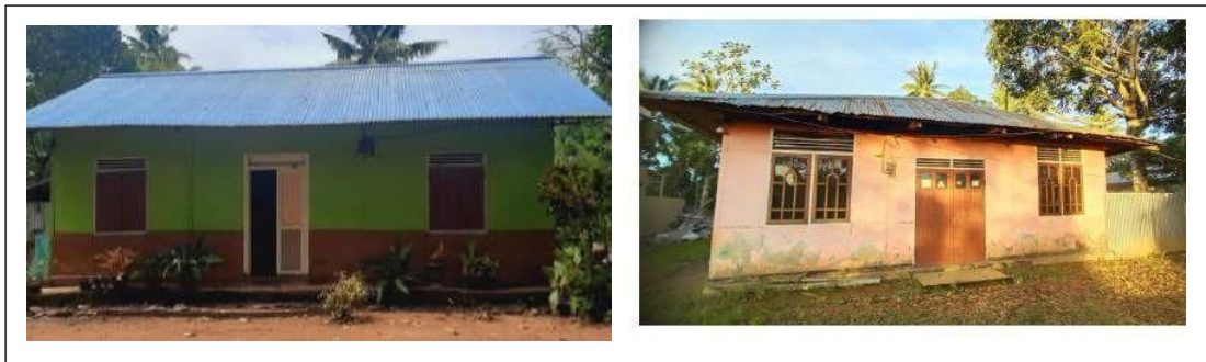
Figure 2 The Roof Shape of Rumah Kancingan around 1950s on the left and 1980s on the right
