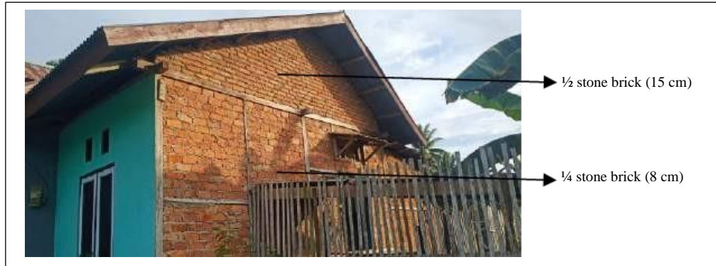
Figure 4 Brick masonry construction on the open gable roof shape of Kancingan houses
